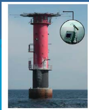
Fig. 1. Picture of the Gustaf Dalin Lighthouse Tower (GDLT) in the northern Baltic. Inset of the Swedish coast. The inset displays a picture of the SeaPRISM above-water autonomous radiometer installed on the tower.
